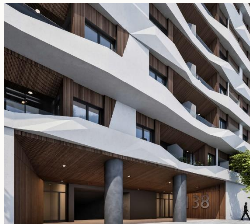
Home2 Suites by Hilton Madrid Retiro** (Opening 2028)
